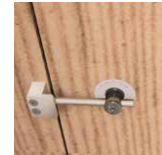
F. Lever lock (Internal view)
